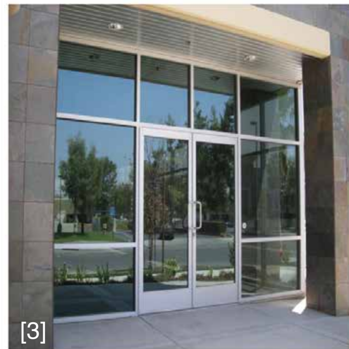
Standard aluminum glazed storefront doors - Simple and clean look - CMH outswing doors - keep a similar aesthetic - Key card activated doors to enter living areas - Doors to the vestibule do not require key card activation for easy exit - Accessibility door buttons for accessible access
