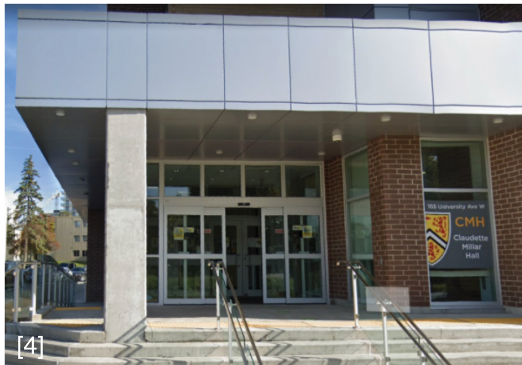
Standard aluminum glazed storefront doors - Simple and clean look - CMH outswing doors - keep a similar aesthetic - Key card activated doors to enter living areas - Doors to the vestibule do not require key card activation for easy exit - Accessibility door buttons for accessible access
