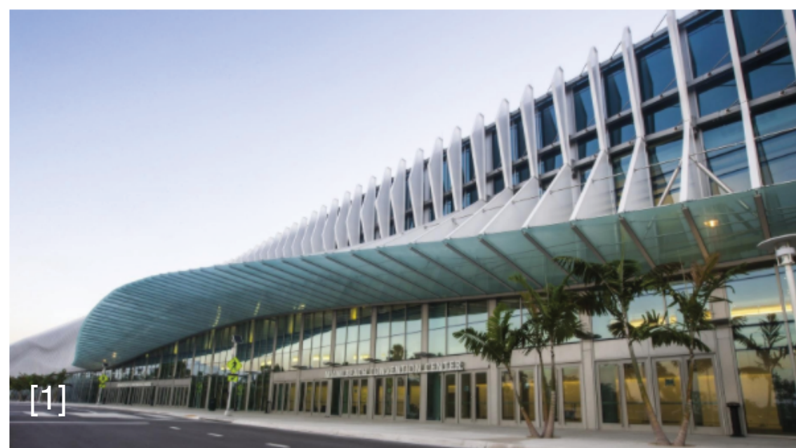
Miami Beach Convention Center, Miami USA - Cantilevered Fins extruding out of the building indicate entrances - Glass Panels under fins to protect from rain and provide shading - Parametric fins and canopy resemble a wave-like pattern - Fin design attach to curtain wall
